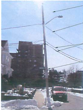
EXISTING CONDITIONS PHOTO DETAIL
