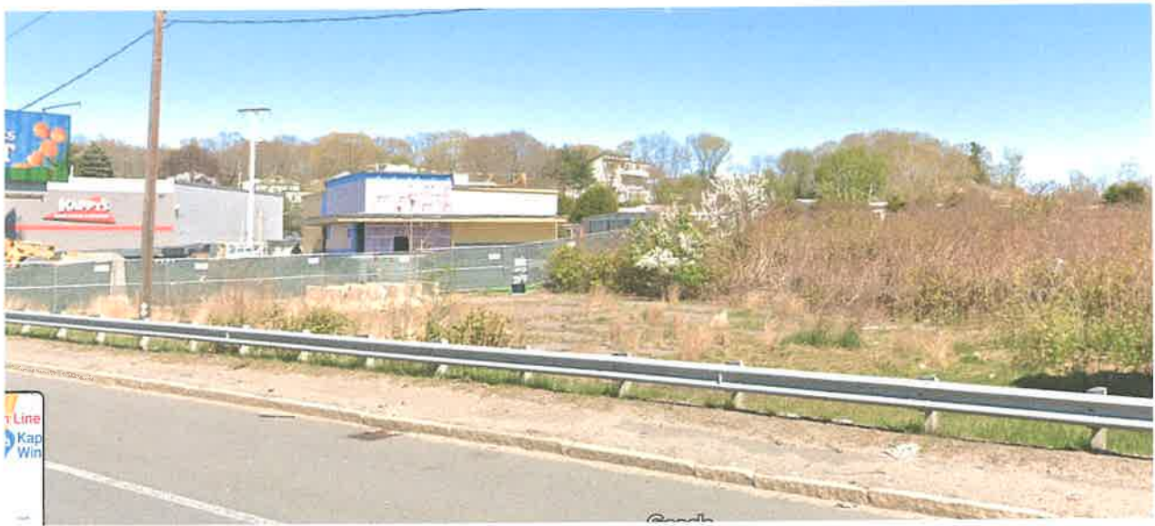
Looking from South
