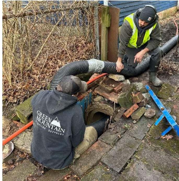
Green Mountain's Crew Cleaning Drain Pipe on Constance St.
