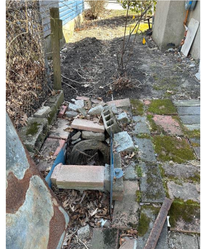
Drain Inlet at 22 Constance St.
