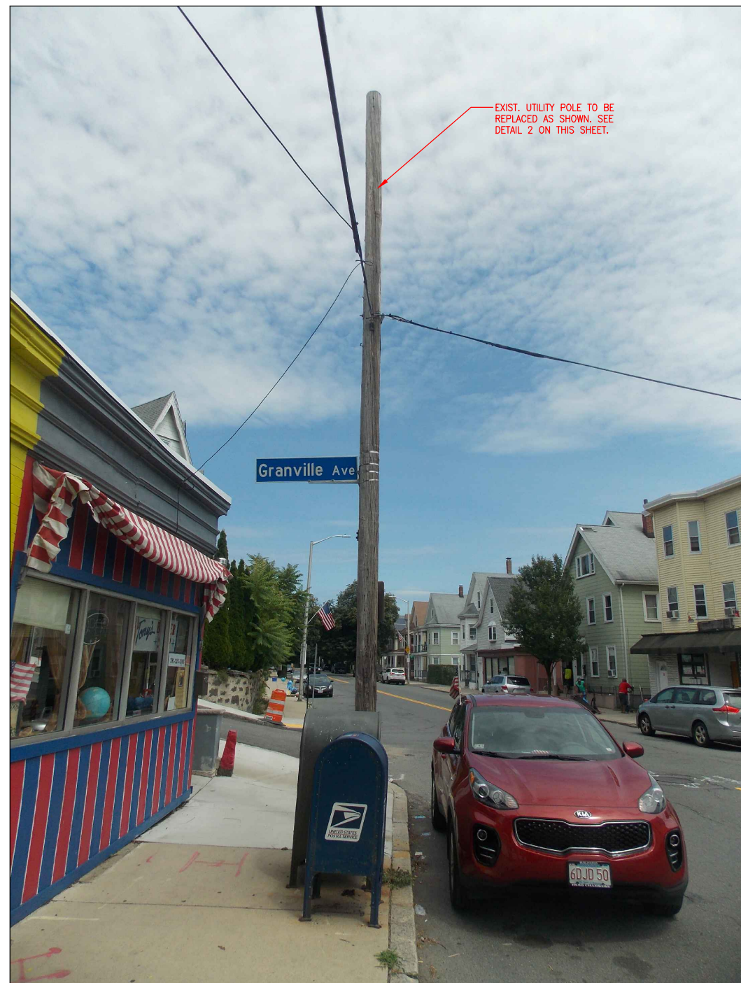
UTILITY POLE #246/64 PHOTOGRAPH (EXISTING CONDITIONS)
