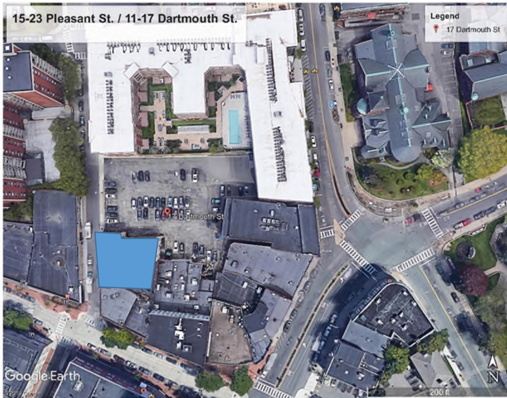
1. Aerial Image of site (Google Maps 2020). Building in blue to be demolished.
