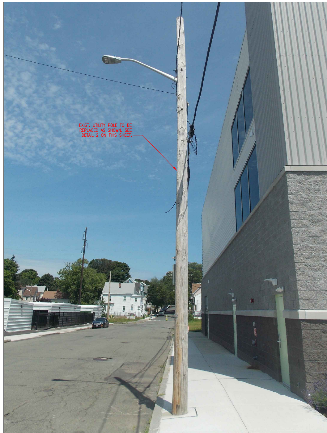
UTILITY POLE #4842 PHOTOGRAPH (EXISTING CONDITIONS) SCALE: NO SCALE
