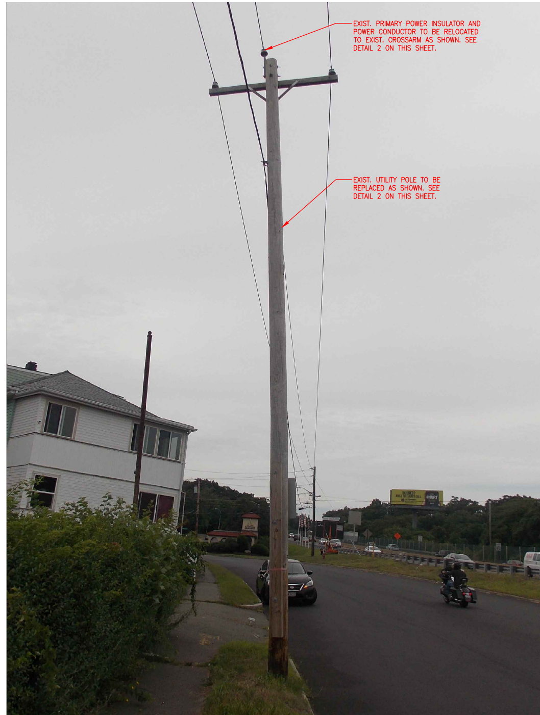
UTILITY POLE #1 PHOTOGRAPH (EXISTING CONDITIONS) SCALE: NO SCALE
