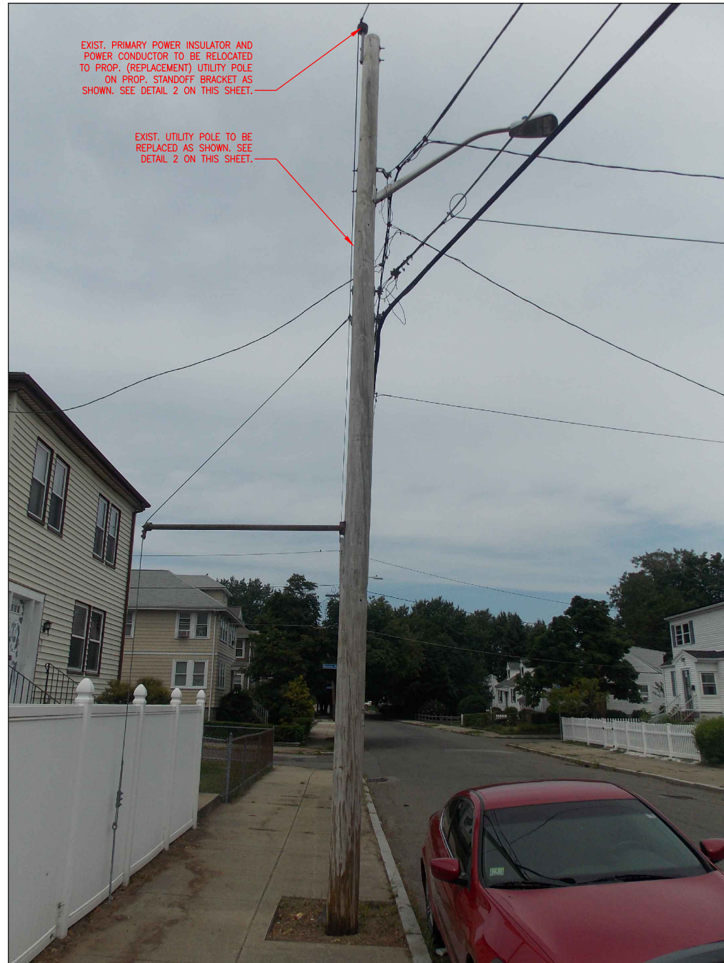
UTILITY POLE #2138 PHOTOGRAPH (EXISTING CONDITIONS)
