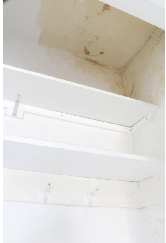
Image 30 Water damage in ceiling of closet of northeast room, below chimney with large crack.
