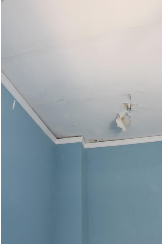
Image 29 Water damage in ceiling of northwest room, below chimney with large crack.
