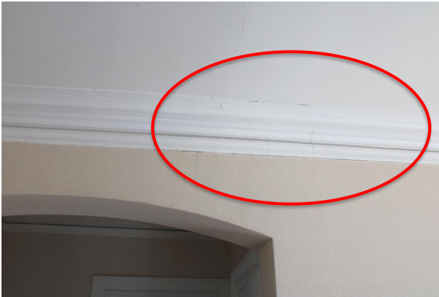
Image 27 View of cornice, second floor stair hall, looking south. Note cracking and irregularity of finish at this location. Same condition is observed at opposite end of stair hall.
