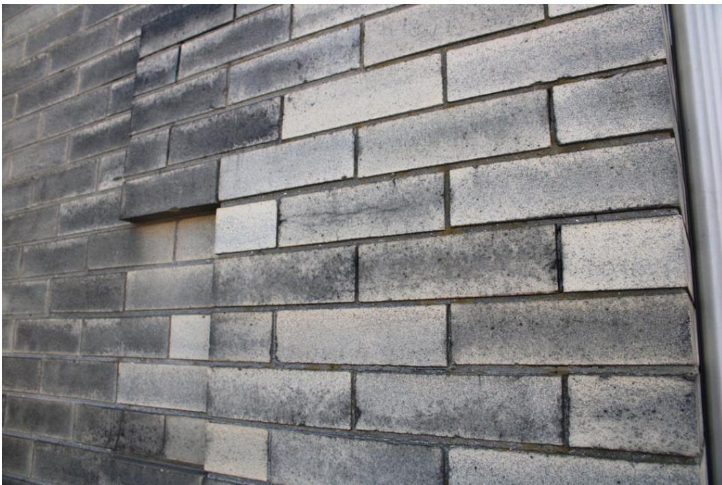
Image 3 Typical brick conditions showing heavily stained bricks, narrow, recessed mortar joints.
