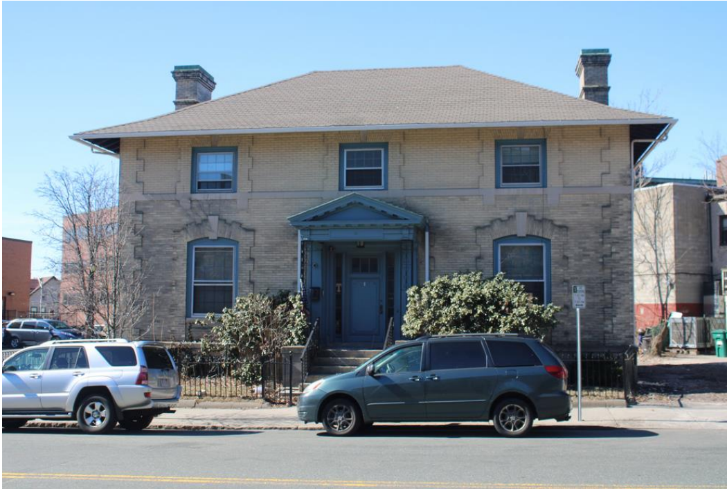
Image 1 East elevation. Note brick treatment around windows and at corners as well as extensive soiling at the corners and below the second-floor level.
