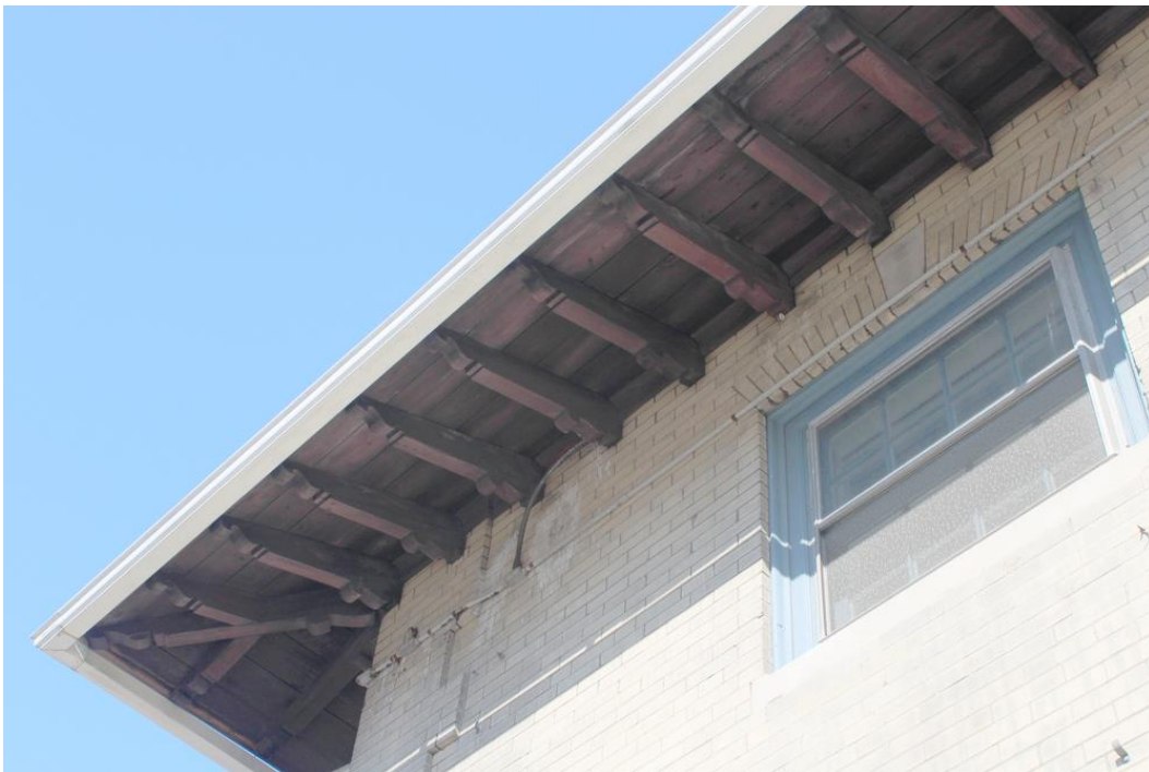
Image 15 View of roof overhang showing original rafter tails.
