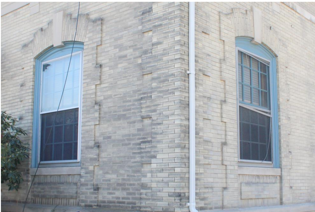
Image 12 First floor windows, northeast corner. Window at right has damaged exterior storm window.
