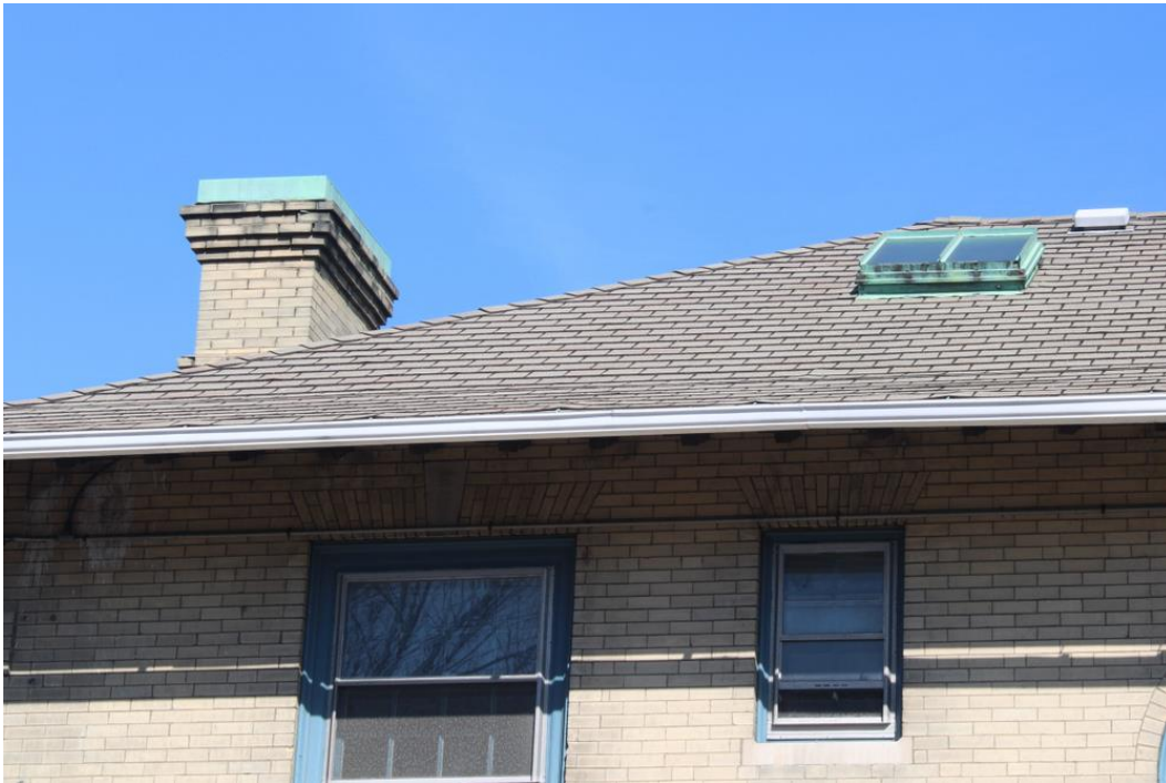
Image 14 View of roof showing asphalt shingles and original skylight for attic space.
