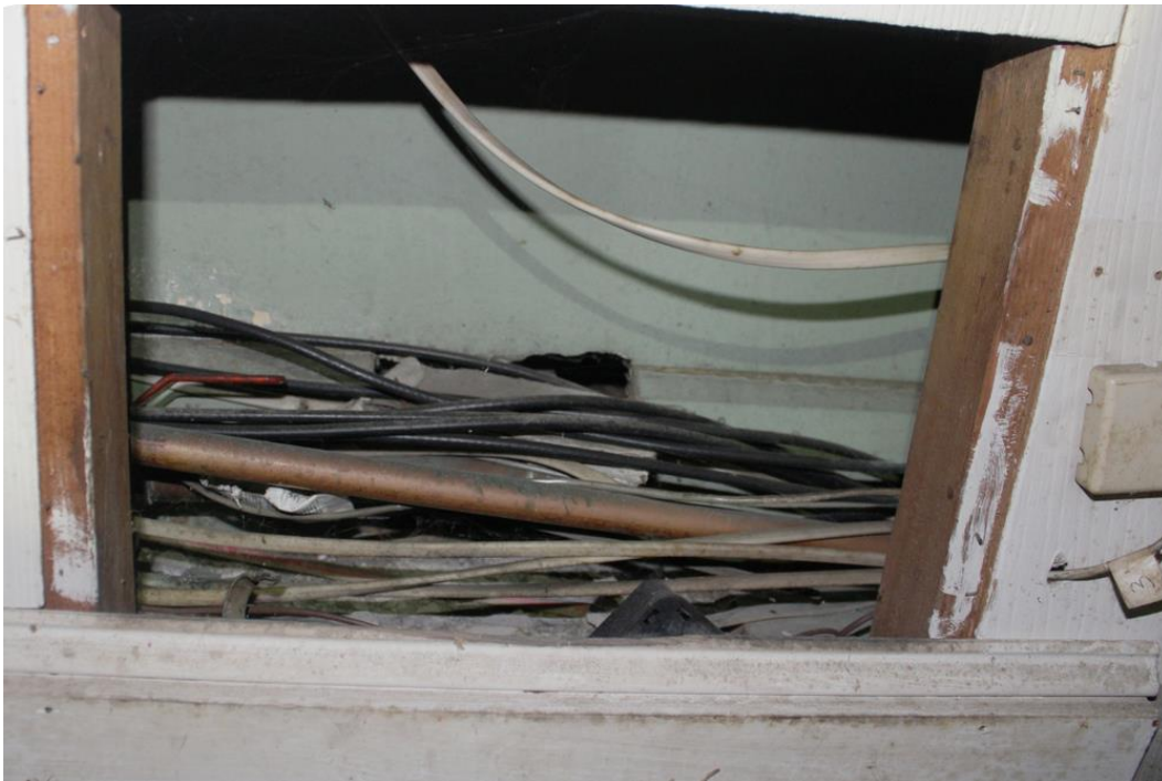
Image 26 View in wall opening showing original painted plaster wall and small section of wood baseboard trim. Details suggest an original level of finish to the basement space.
