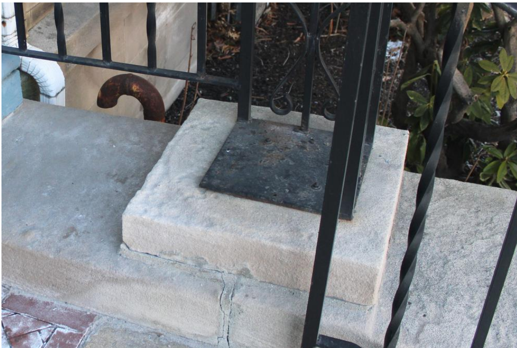
Image 11 Circular outline of original wood column, granite base at front portico.
