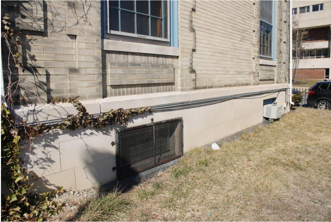
Image 5 South elevation showing limestone foundation with limestone water table.
