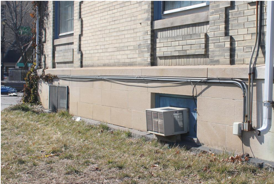
Image 13 Basement window openings showing either original metal grille work or modern air conditioning unit fit into plywood opening.
