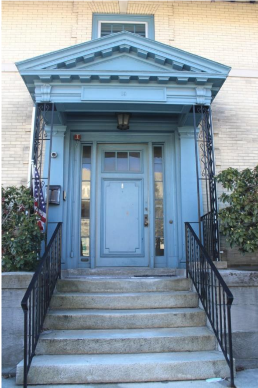
Image 7 Front entrance and portico. Iron supports are not original. All other elements including the postal slot and the light fixture appear to be original.
