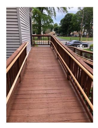
Wheelchair ramp from two angles showing newly installed handrails.
